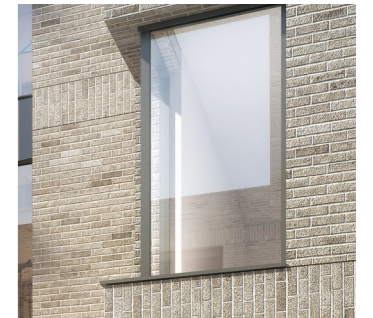
Solider course brick banding denoting floors
