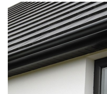
Soffit & Fascia detail
