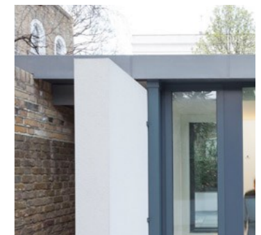
Soffit & Fascia detail
