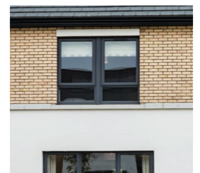
Plaster window detail
