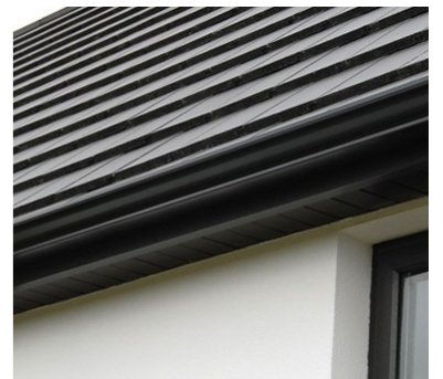
Soffit & Fascia detail
